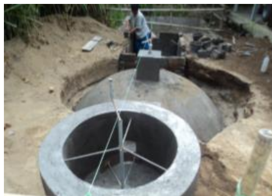
Figure 10. Biogas Construction with Community Participation
