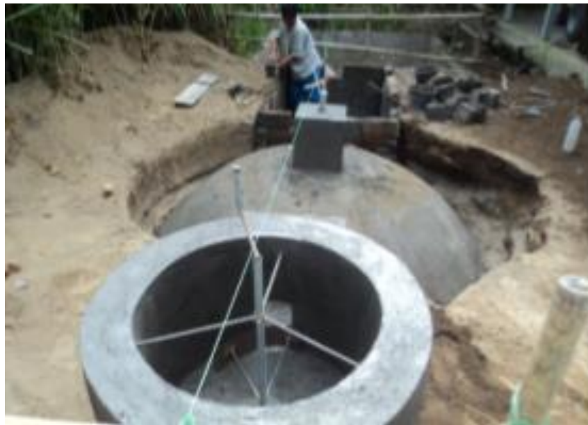
Figure 9. Biogas Construction with Community Participation
